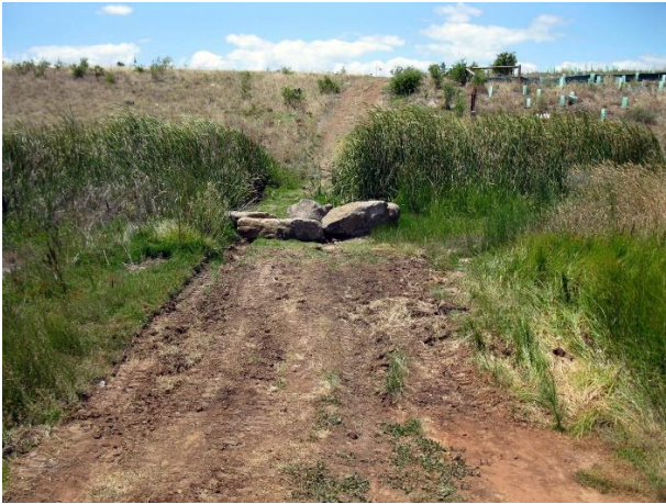
After: Melbourne Water responded quickly, the mess was cleaned up and a barrier of large rocks was installed to prevent vehicle access
